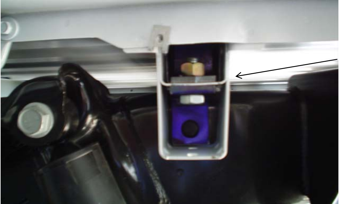
INSTALLATION OF BRACKETS SHOWN. READY TO DRILL HOLE.
